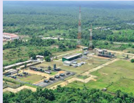
Aerial View of Facilities
