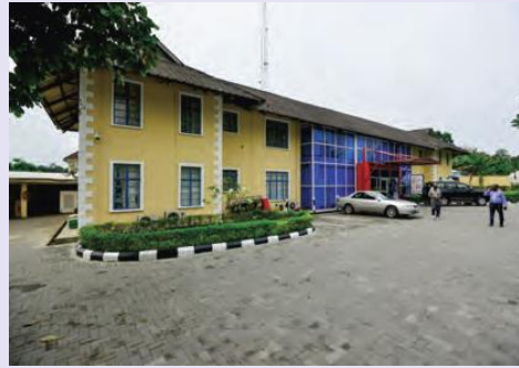
SEPLAT Base Office, Sapele
