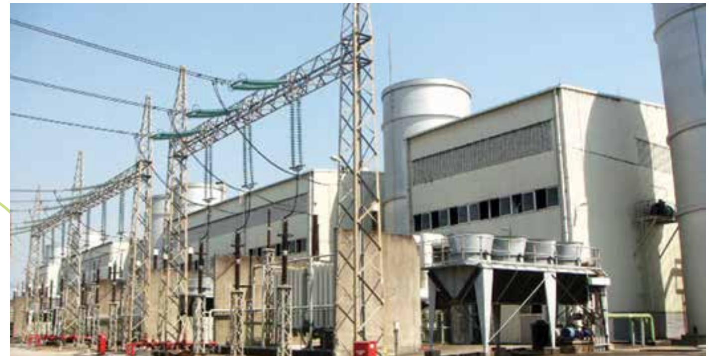
Ughelli power plant rehabilitated
