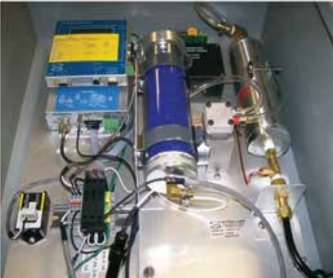
Automated Flood Early Warning Systems
