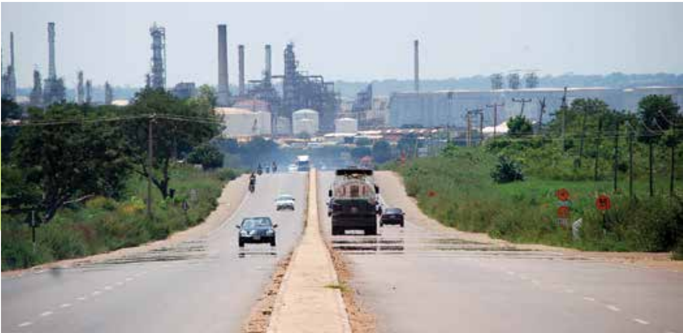
Rehabilitated Refinery Access Road in Kaduna, Kaduna State
