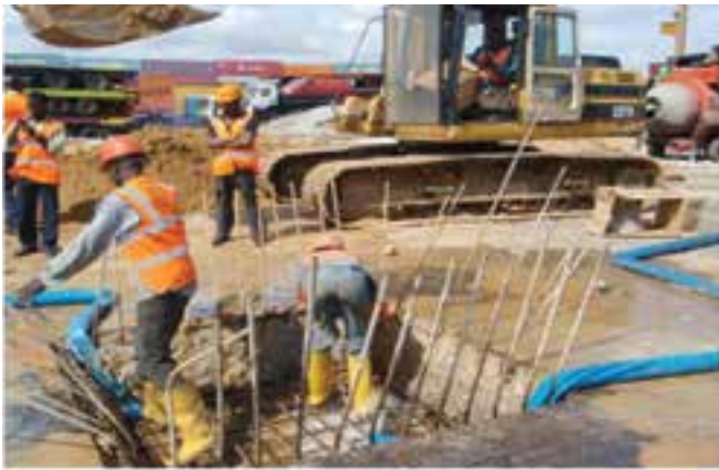
Rehabilitation of Quay Wall and Quay Apron at Tinian Island port
