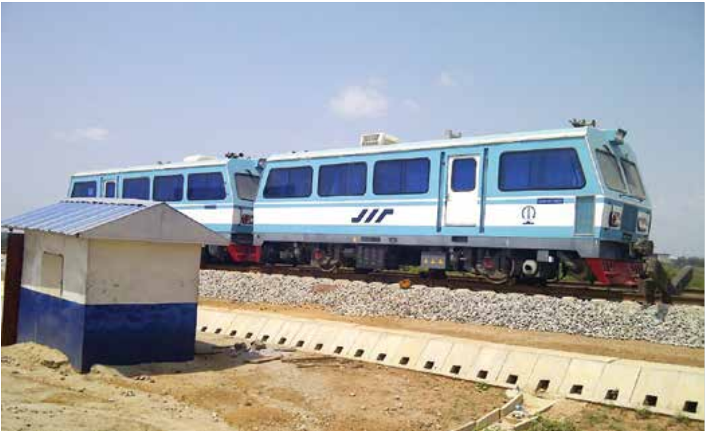
Test Wagon running on the advanced Abuja Metro Line under construction
