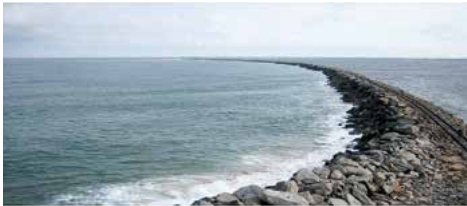
East west mole / breakwaters, Lagos
