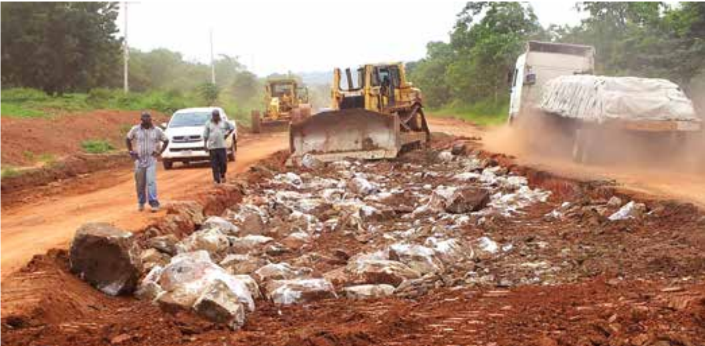
Rehabilitation of Ayangba-Ajaokuta road in Kogi State
