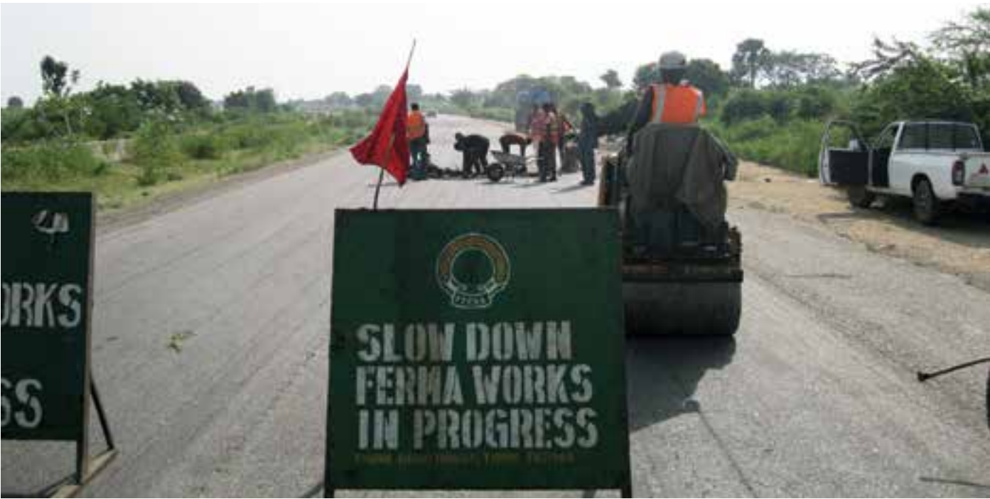
Repairs works on Kano-Kaduna expressway by FERMA
