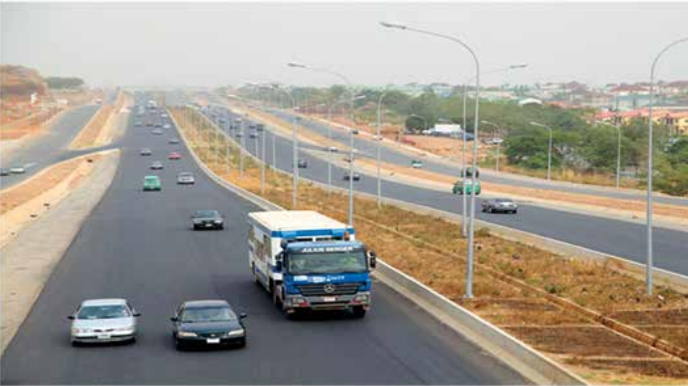
The 10-lane Airport road under construction
