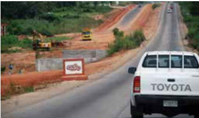
Ongoing Abuja-Abaji road dualization
