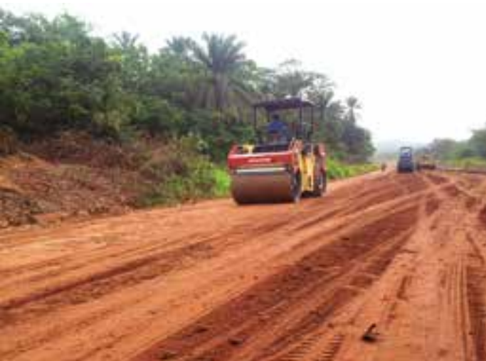
Construction of Nsukka-Obollo-Ikem-Nkalagu road in Enugu and Ebonyi States
