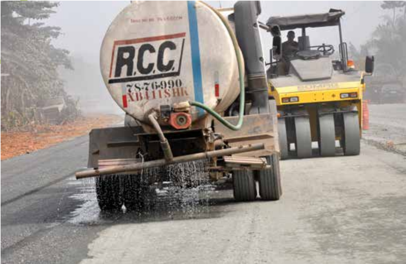
Ongoing work on Benin-Ore-Shagamu-Lagos expressway
