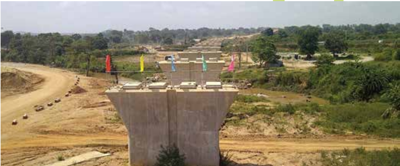
Concrete pillars for Abuja metro line project fast progressing
