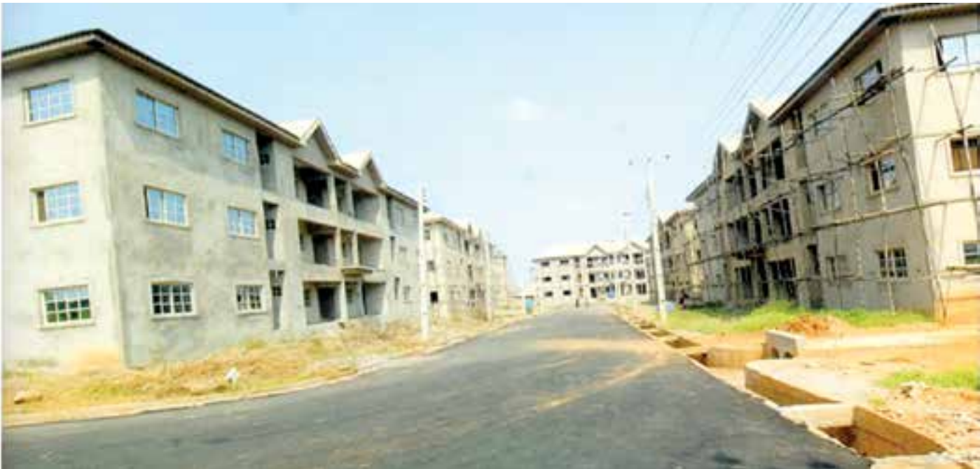
On-going Federal Housing Authority Project at Abesan, Lagos State
