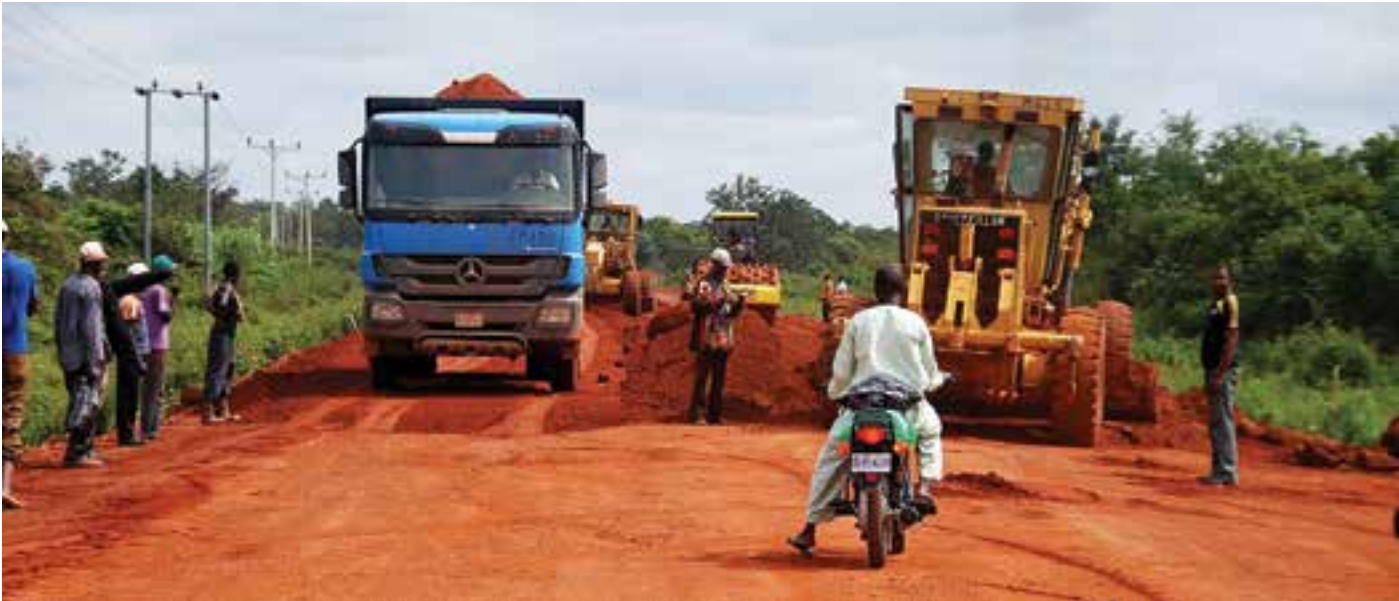
Rehabilitation Of Lafia-Obi-Awe-Tunga Road in Nassarawa State
