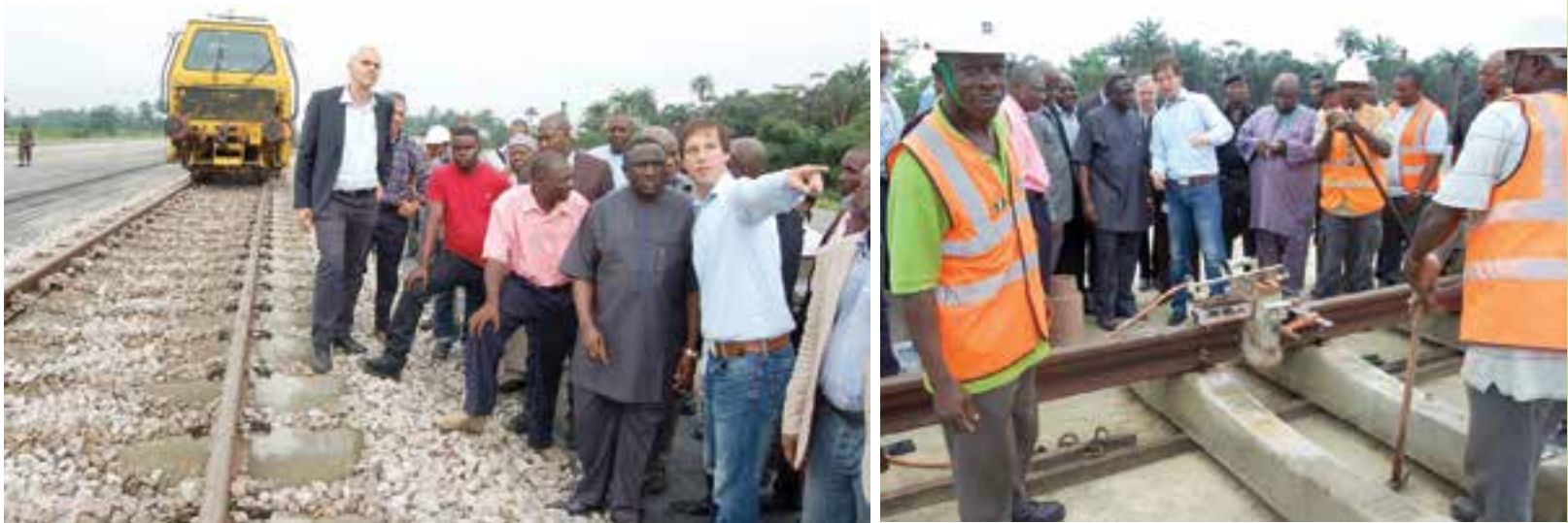
Hon. Minister of Transport, Alhaji Idris Umar, inspecting on-going rehabilitation and completion of Itakpe-Ajaokuta-Warri standard gauge rail line
