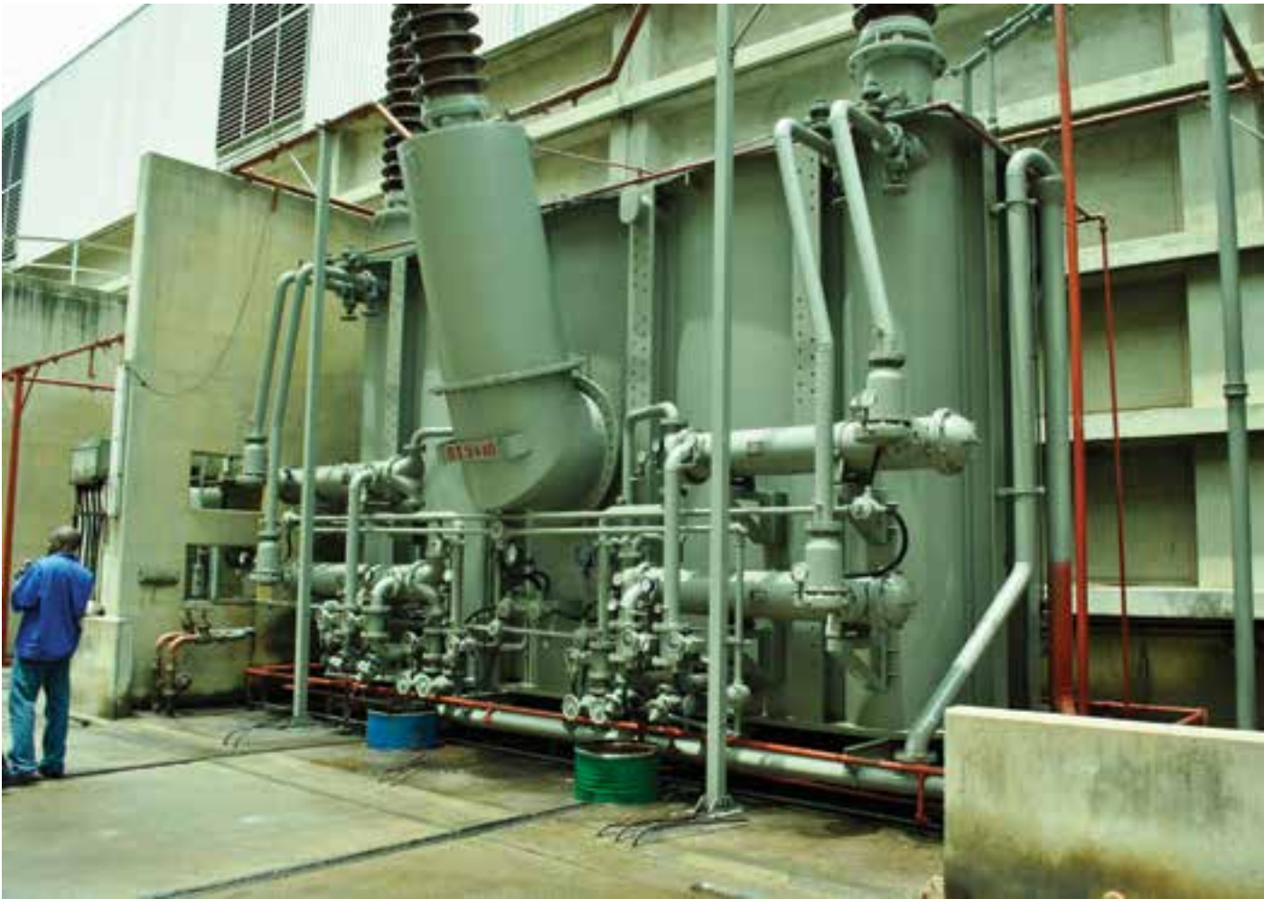
Kainji power plant rehabilitated
