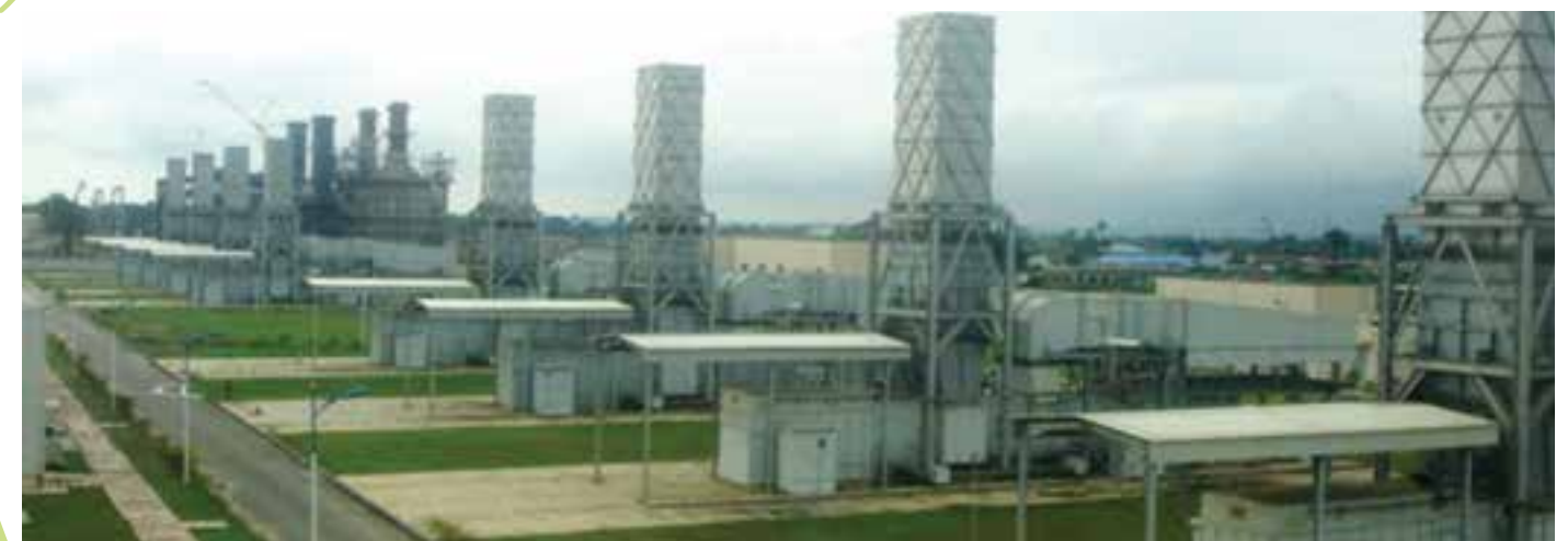
Olorunsogo power plant rehabilitated
