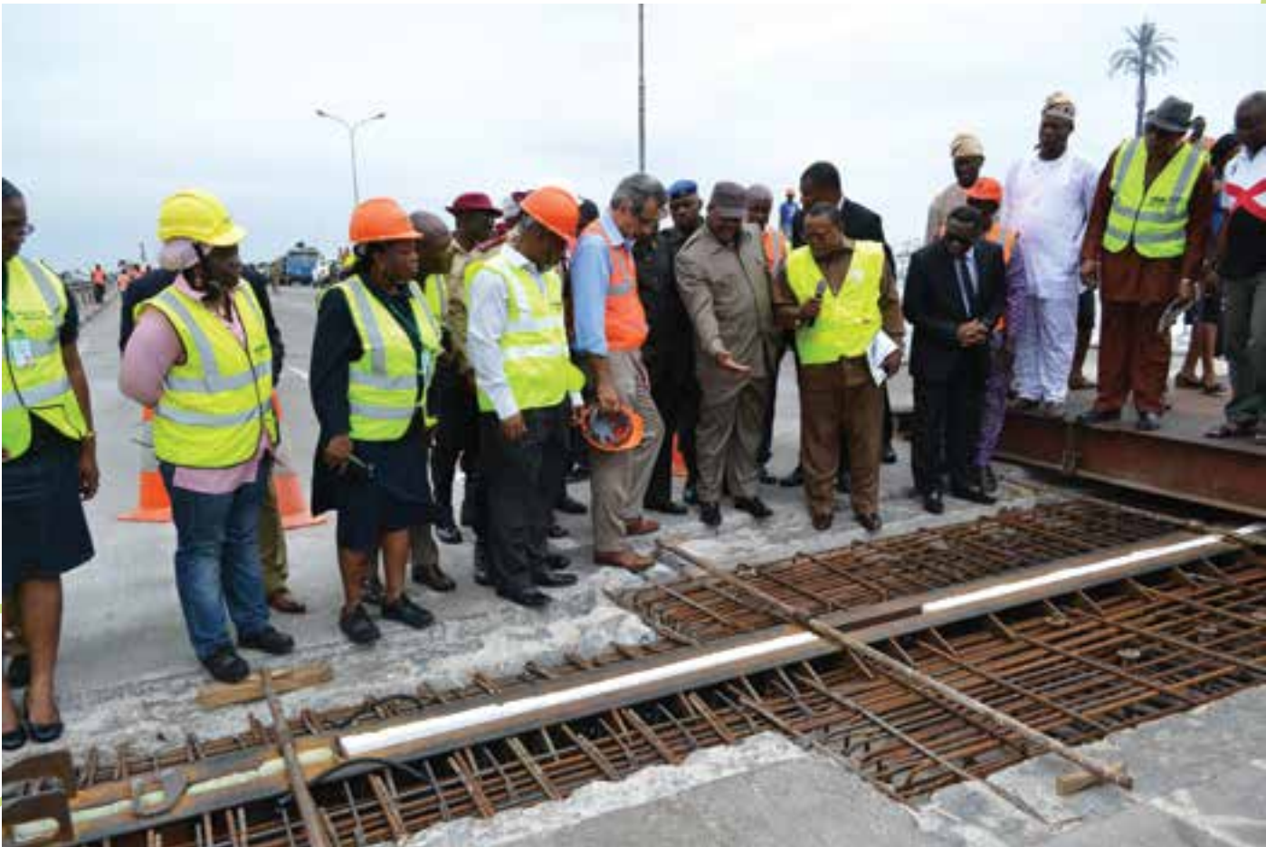
Minsiter inspecting repair work currently on 3rd Mainland Bridge
