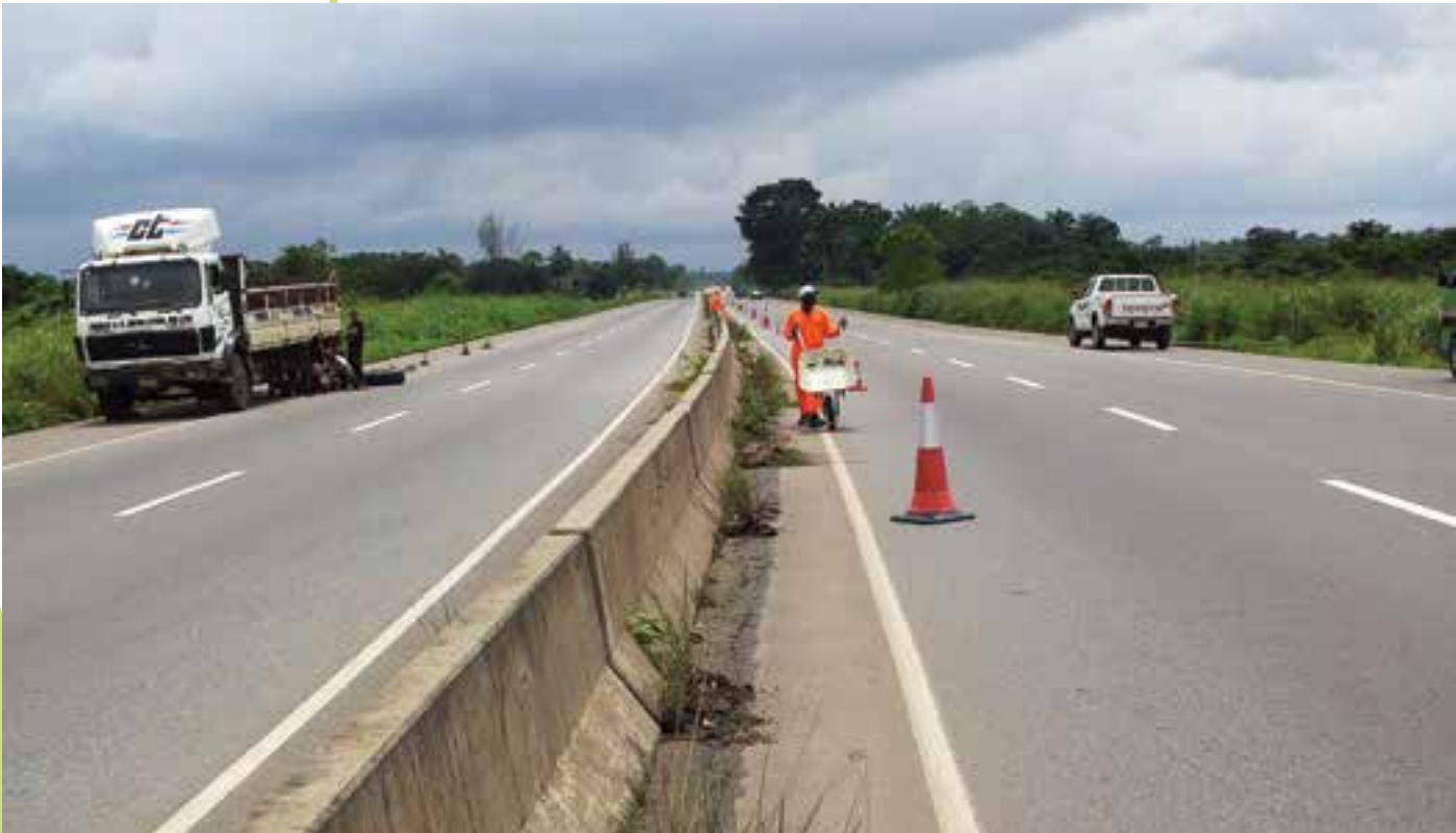
Newly completed Dualized Onitsha-Owerri expressway in Anambra and Imo States
