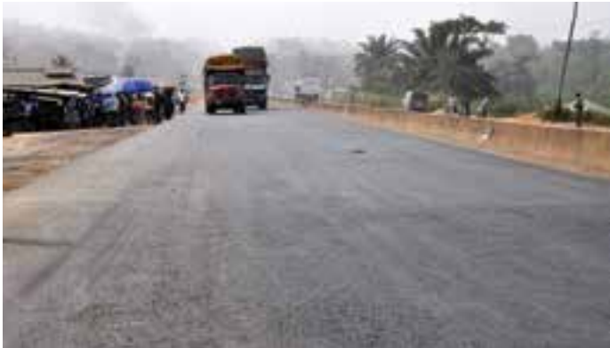
Completed section of Benin-Ore-Shagamu-Lagos expressway
