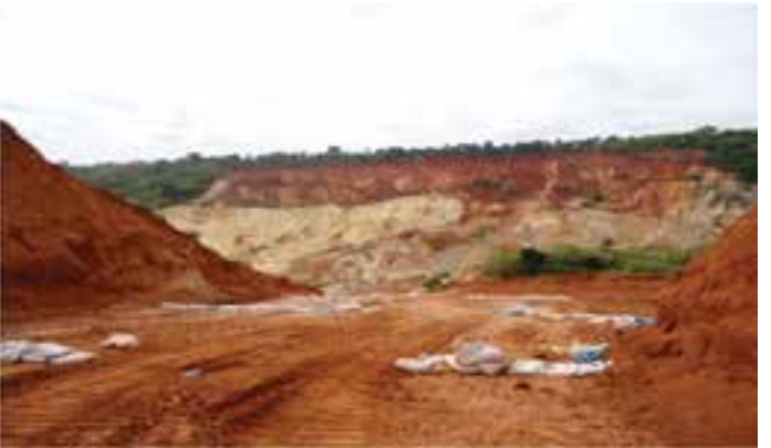
Erosion Challenge in Auchi (Before intervention)
