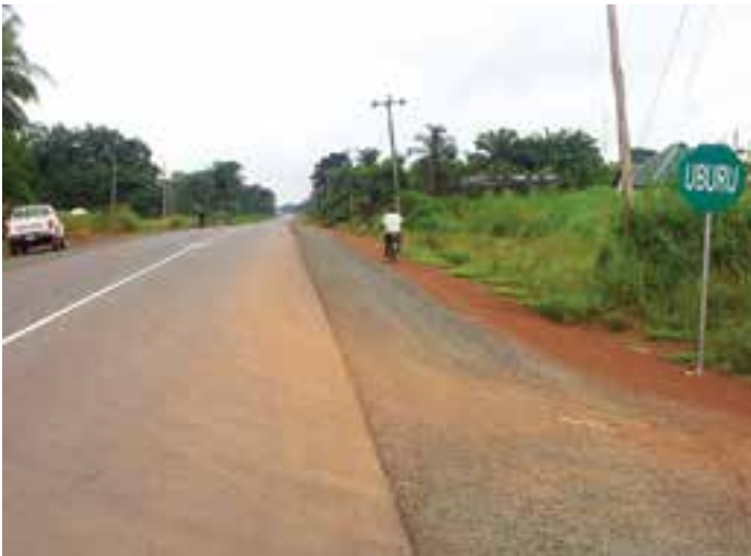
Newly completed Obiozora-Ishiagu-Enugu state Border road in Ebonyi State
