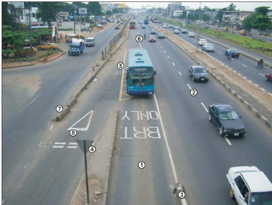
BRT Lane: Typical Merge/Diverge Arrangement
