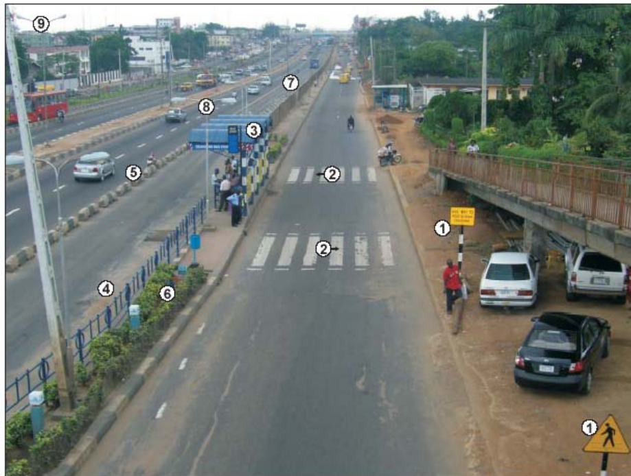
BRT Lane: Typical Merge/Diverge Arrangement
